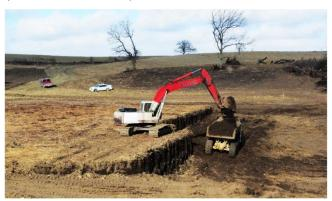
This picture taken in early December of 2017 shows the excavation of nearly 60 years of topsoil, up to nine feet deep, within the structure pool area.
