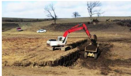
This picture taken in early December of 2017 shows the excavation of nearly 60 years of top soil, up to nine feet deep, within the structure pool area.
